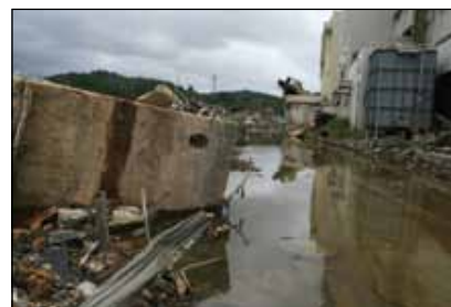
Plate 8: (A – top) Flooding in an area near the coastline due to land subsidence (photo taken in Minami-sanriku), (B – bottom) and a road underwater (photo taken in Ishinomaki).
